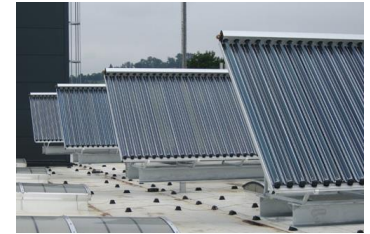
Evacuated Tube Collectors
