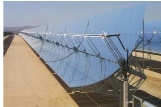
Parabolic Trough Collector
